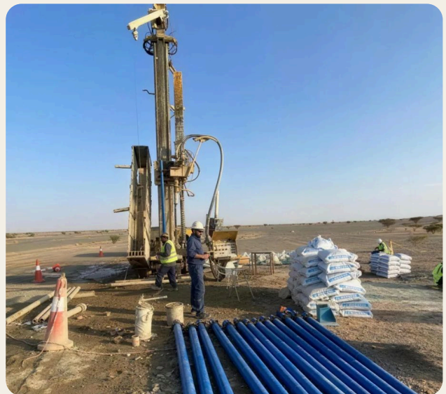
Monitoring-well installation
