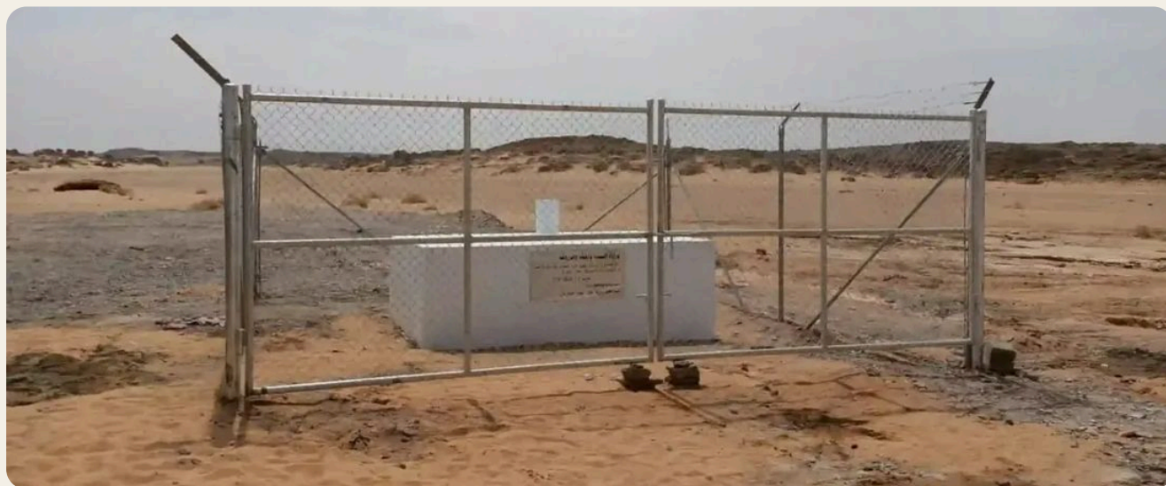
A protected groundwater monitoring well
